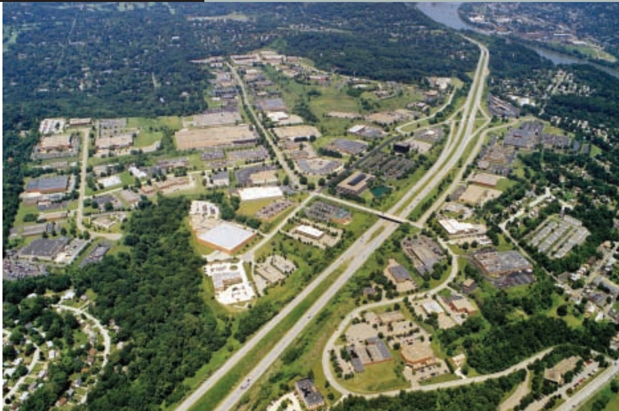
The original RIDC Industrial Park in O'Hara Township still contains roughly a dozen buildings owned by the RIDC.
